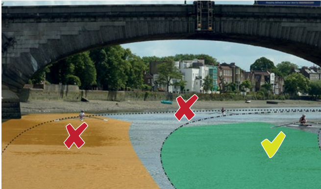
Looking downriver at Kew Stone Bridge centre arch from the Fairway
